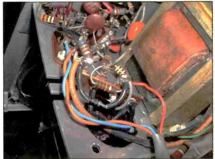
Photo E. A four-position terminal was installed using one of the old filter capacitor's mounting holes. The new radial lead filter caps and the 1N4007 silicon diode are mounted on the strip.
