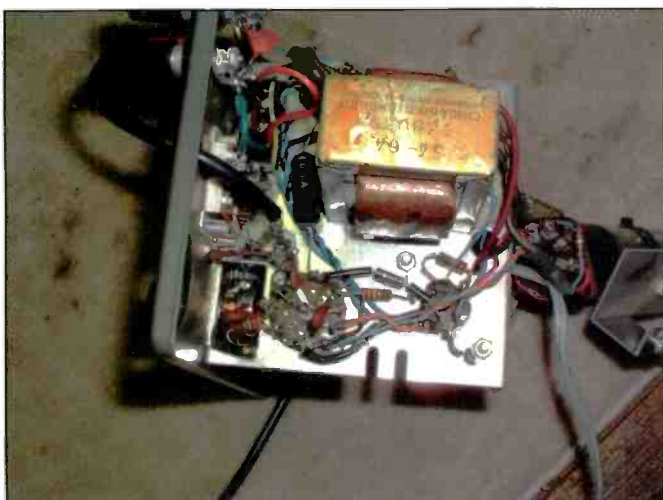
Photo D. This is a view showing where the original can filter capacitor was mounted.
